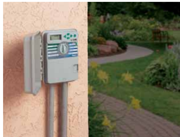
An automatic controller stores information on what days to water, what time to start watering and how long each zone will run.
