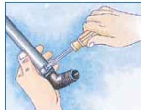
Poly Pipe: 2. Tighten clamp around pipe and fitting.
