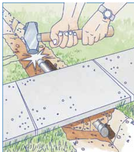
Connect pipe under a walk or driveway by capping off the ends of galvanized pipe and "hammering" through.
